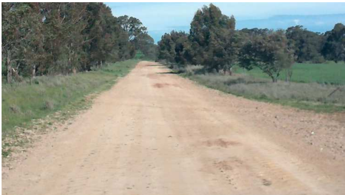
Typical Class 3a Rural Sheeted Road showing signs of wear in patches
