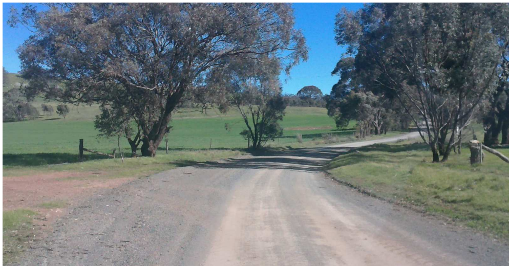
Typical Class 2b Rural Sheeted Road with exposed subgrade
